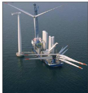
Offshore windmill installation jackup system(2011) 100 DA hydraulic cylinders 650 bore x 320 rod x 2300 mm stroke
